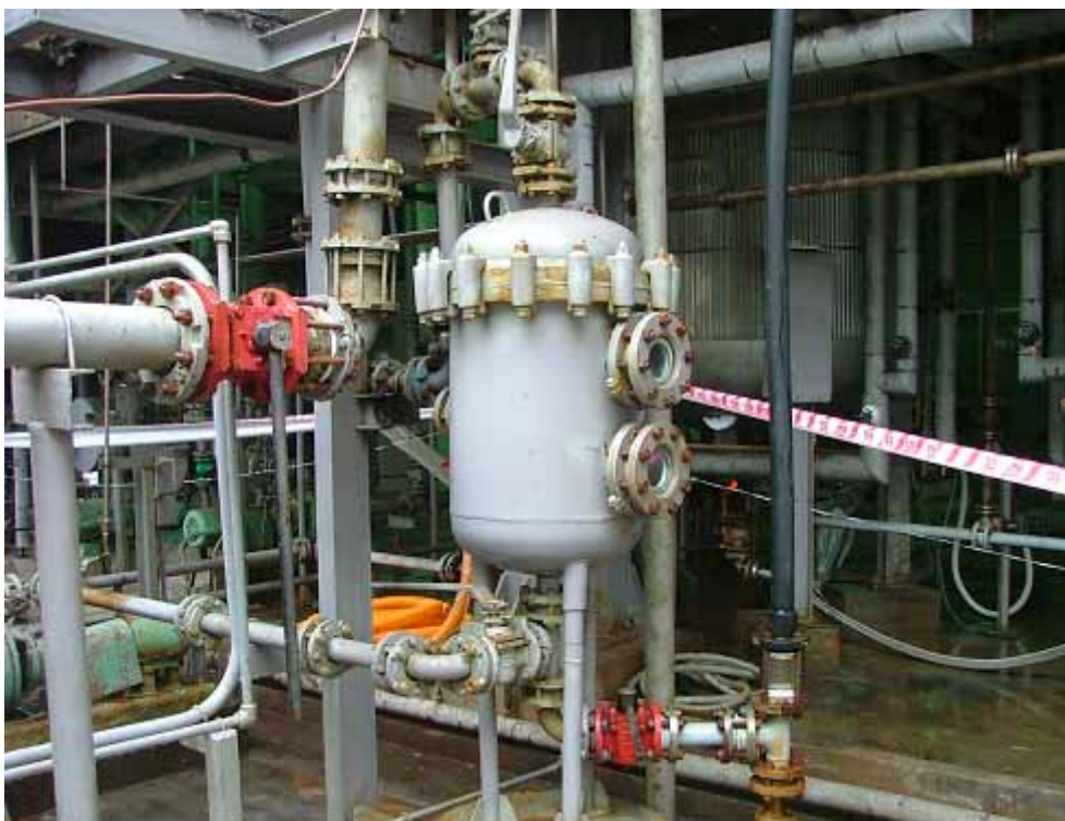
Fig. 3: Phase Separator
