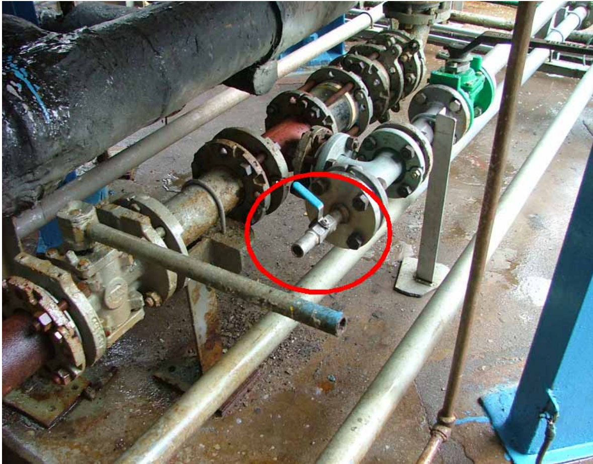
Figure 1: HCL released sampling valve (3/4", Ball valve)
