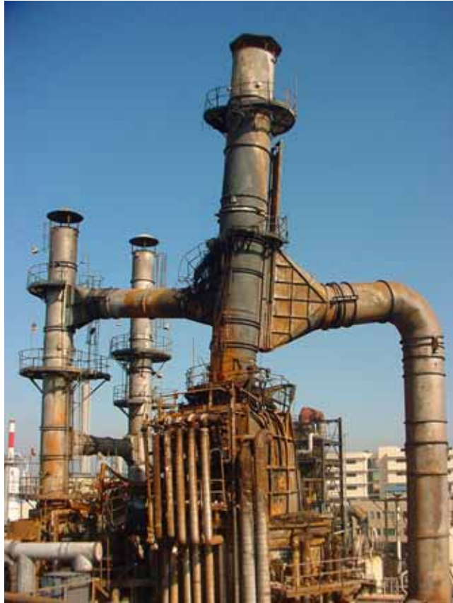
Fig. 7 : Appearance of the Reboiler Heater after Fire
