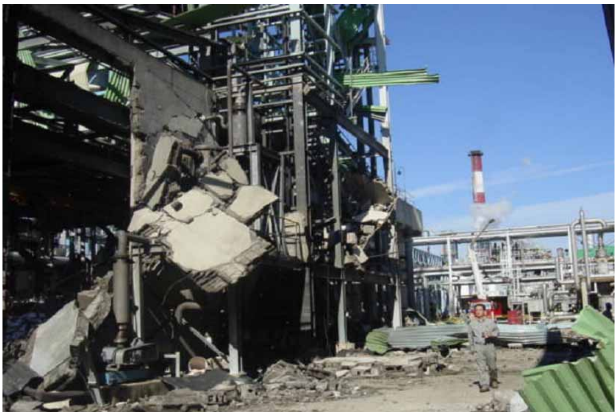
Fig. 1 HDPE Unit after Explosion
