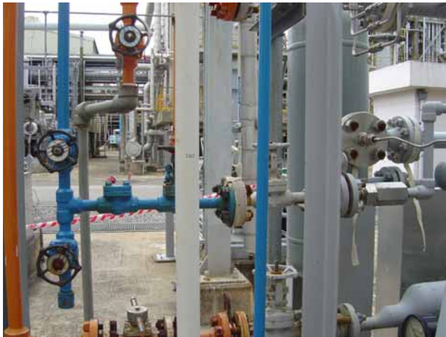
Fig. 4 : Nitrogen purge line of compressor suction part
