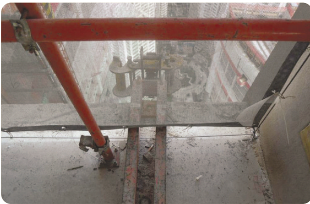
Anchor bolts and brackets in the middle
