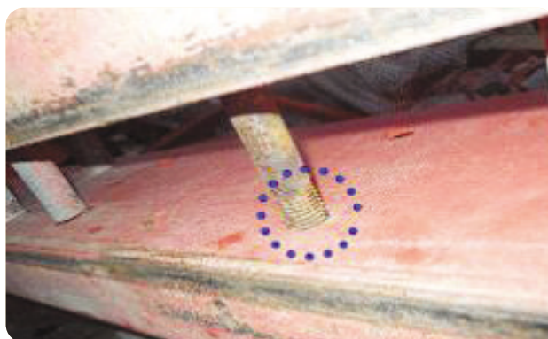
Traces of friction about climbing shoe
