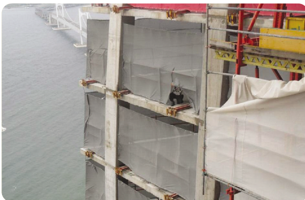
Anchor bolts and brackets in the upper, middle, lower
